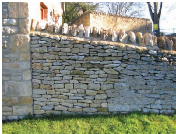
Typical boundary wall, with on edge coping and limited areas of pointing.
